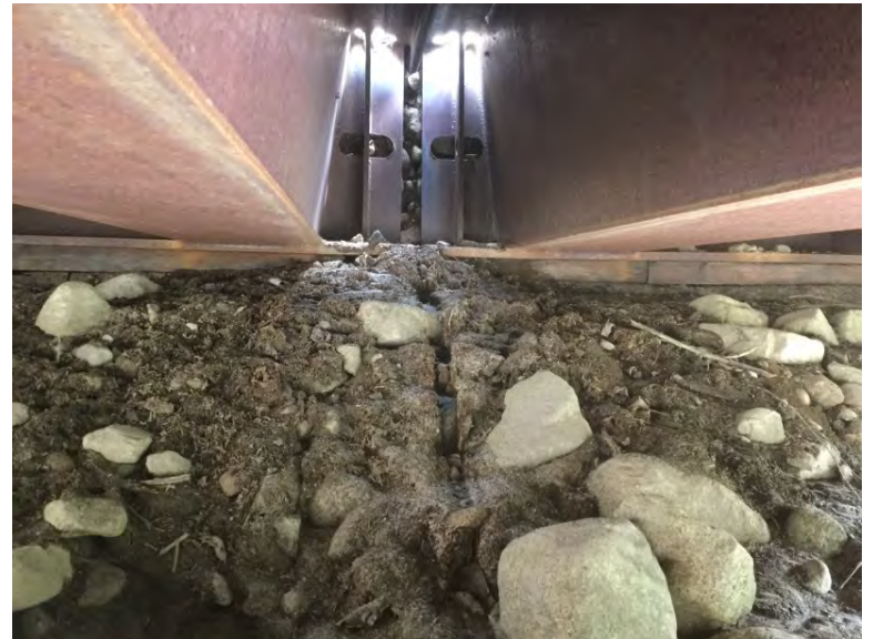
Timber on top of log sill at left bank
