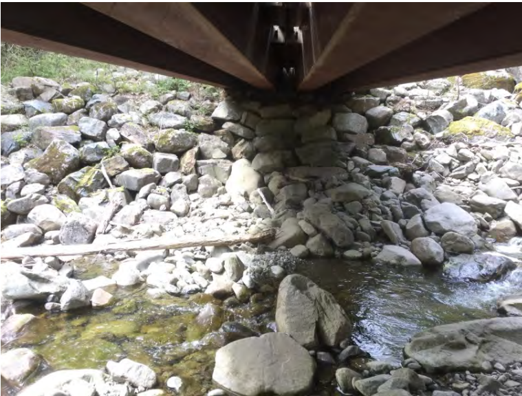
Right Bank Abutment when facing downstream
