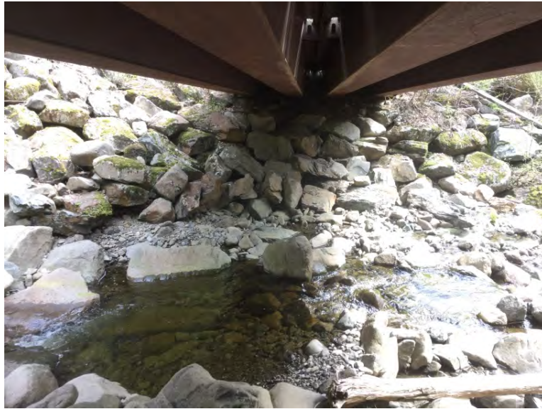
Left Bank Abutment when facing downstream
